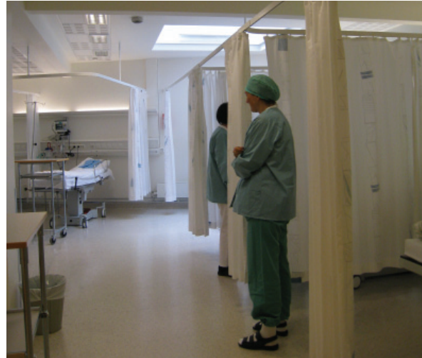
Skylights allowing daylight into patient recovery areas (Burpee, 2008)
